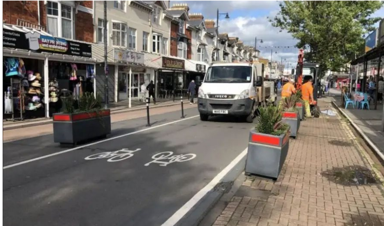
Temporary traffic reduction scheme, 2022.
